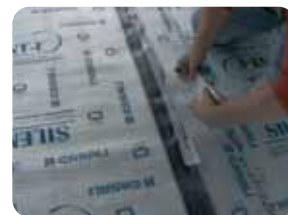
4. Stabilize the membrane by taping the joints
