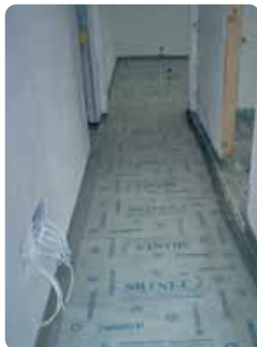
5. Lay the anti-shrinkage net of the regulating slab
