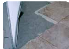
8. Lay the finished floor
