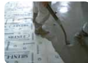
6. Cast the regulation slab
